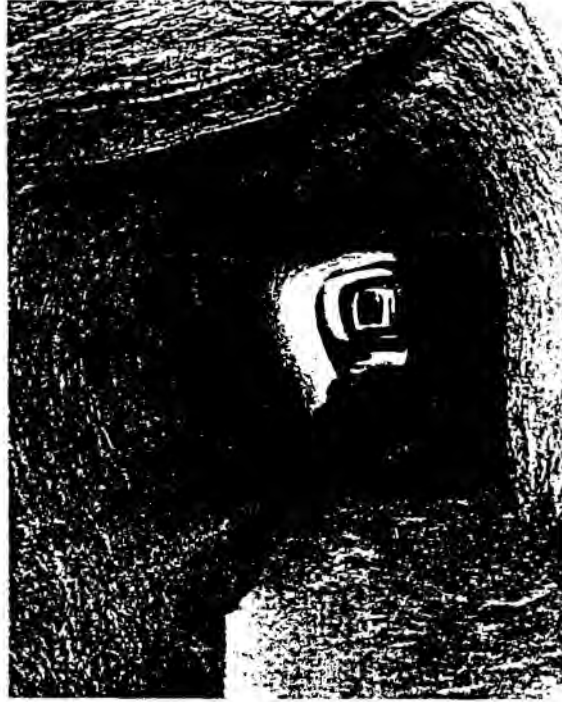
3. Samos: tunnel of Eupalinos The water was carried in a pipeline at the bottom of the trench alongside the left side of the floor of the main tunnel (photo: Deutsche Archäologisches Institut. Athens)
